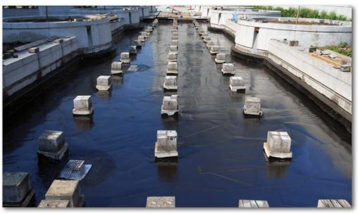
In the paver areas, the TREMproof 250GC would be applied, cured, leak detection was completed and it was ready to be walked on within two days.
