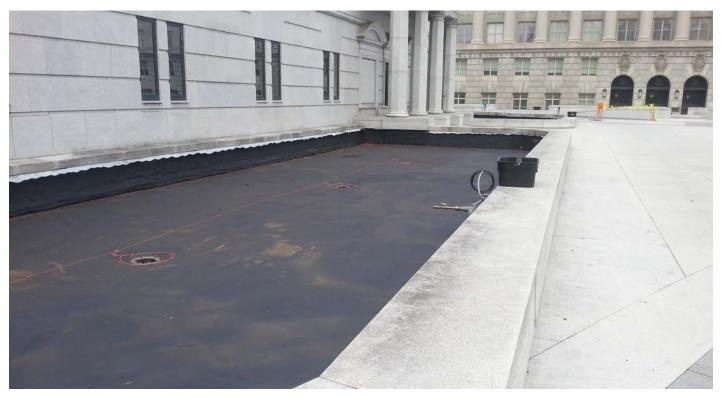
About half of the project included planters and 40,000 square feet of vertical surfaces so the TREMproof 250GC with its trowel-grade version helped to ensure no areas were left untreated or exposed to moisture infiltration. TREMDrain GS drainage mat was used over the membrane to enhance the performance of the waterproofing system by functioning as a water retention layer while designed to also prevent root growth.
