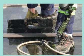
Application of Spectrem 2 sealant on the skylight above the Mayfield Toyota Ice Palace
