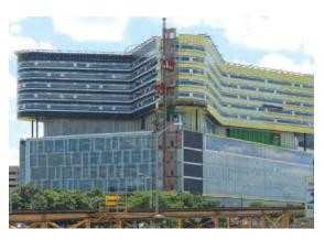
At Rush University Medical Center in Chicago, the building's unique stacking joint design created a challenge. Traditional transitions couldn't pass standard chamber tests. Proglaze ETA provided the flexibility and durability to withstand the expected movement and was able to span the irregular and unsupported floor deflection joints.
